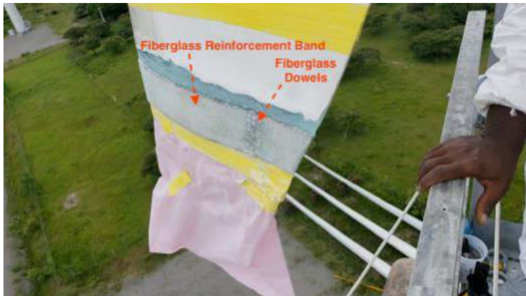
Figure 4.2: Fiberglass bonded in place
