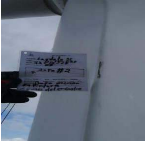
Figure 6.7: T7 Paint flow
