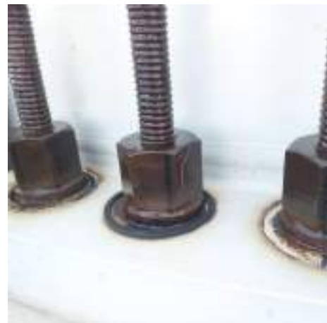
Figure 5.12: Displaced nut
