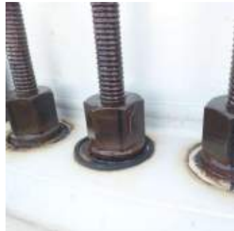
Figure 5.6: Displaced nut
