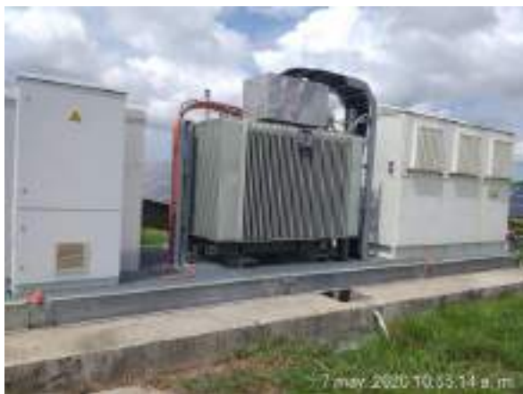
Figure 2.8: Power Block
